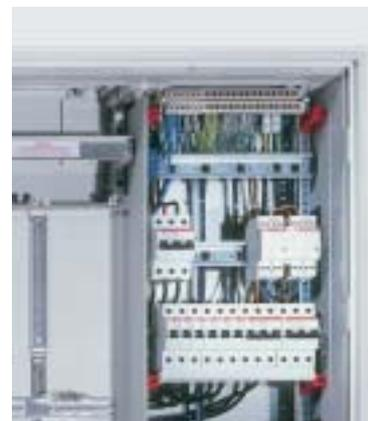
The N/PE Quick busbar can also be installed in **wall cabinets and stand-alone cabinets** in conjunction with the EDF fast installation system.
