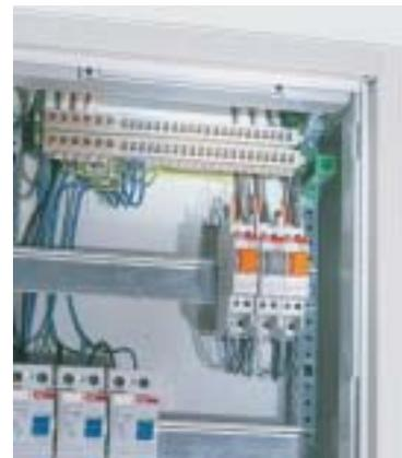
As before, the N/PE Quick busbar can be fitted at different positions in the distributor panels of the **meter cabinet**.
