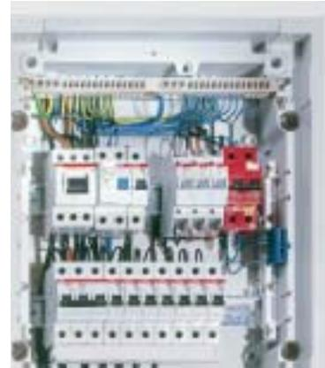
The N/PE Quick busbar is also installed in the usual way in **small distribution boards**.
