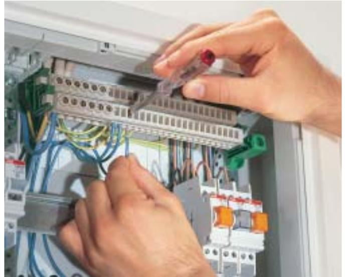
Flexible wires without wire end ferrules are inserted by opening the terminal with a screwdriver. The clamp connection can be released in the same way.
