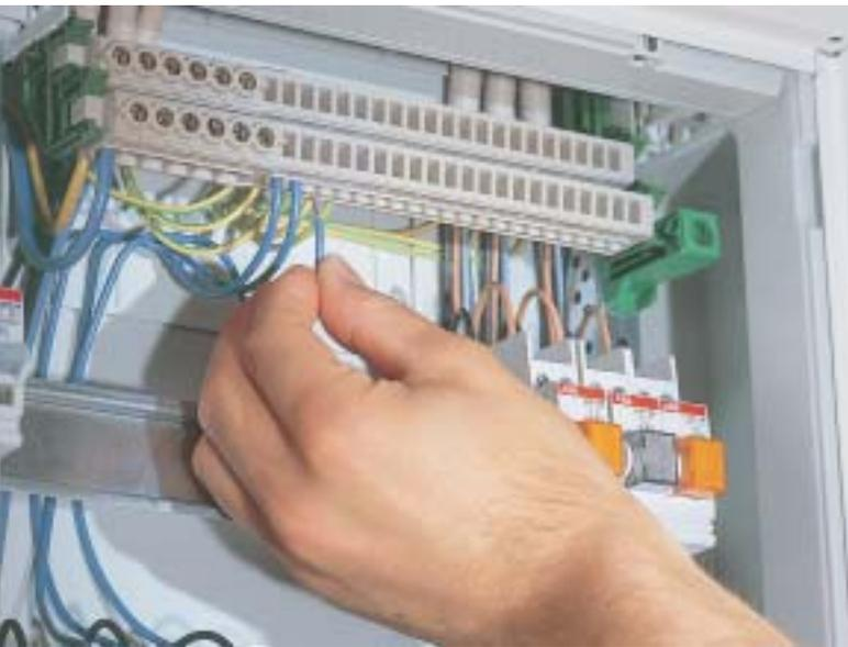
The new connection technology permits the electrician to perform uncomplicated plugging. Rigid wires are simply inserted into the clamping carrier attachment.
